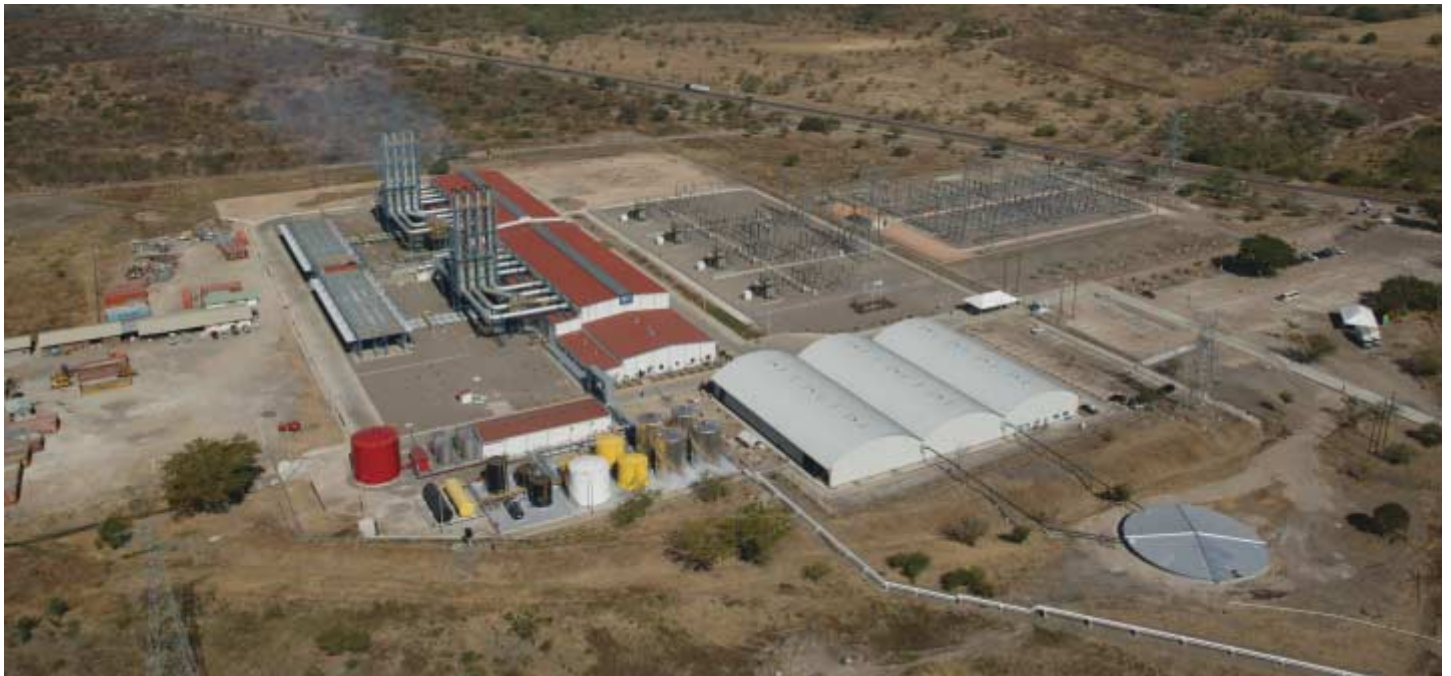
Aerial view of the Pavana III power plant in Honduras.
