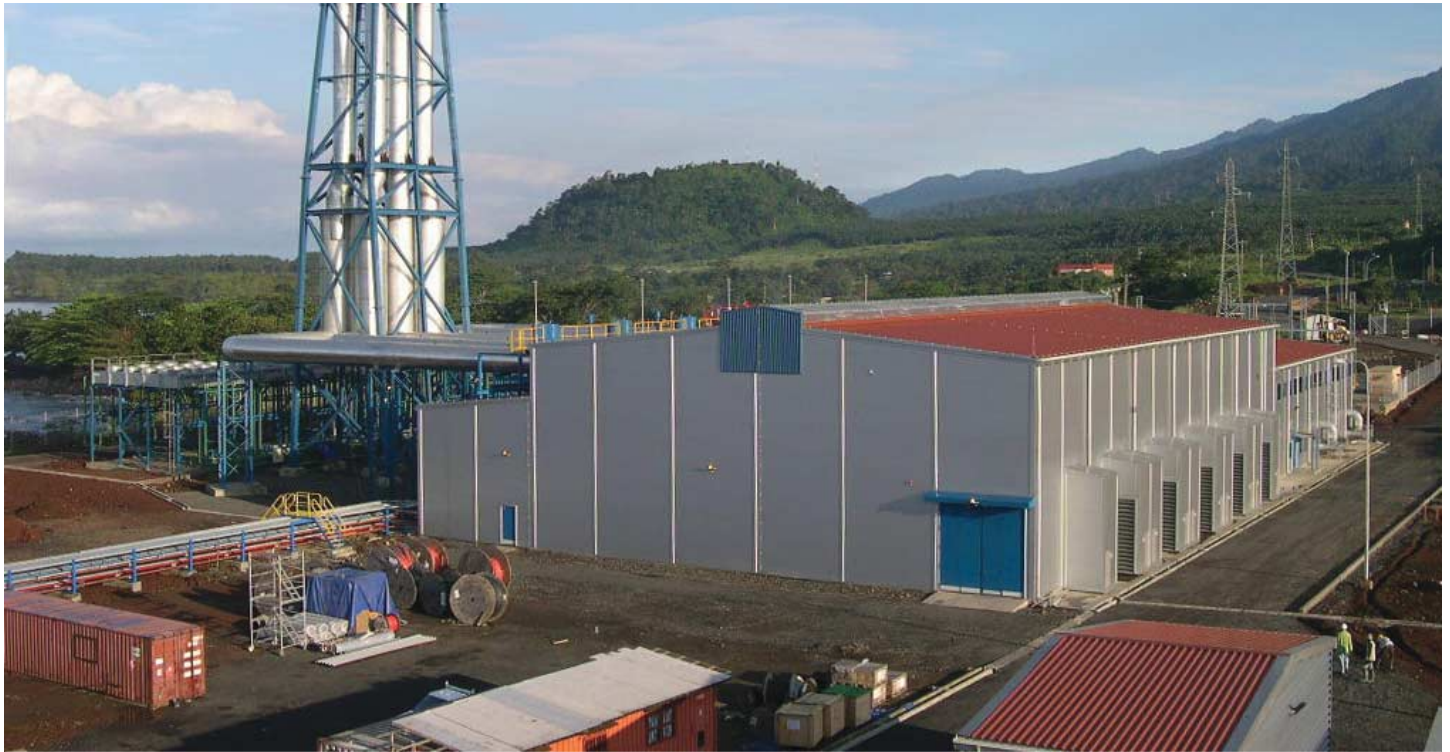
The Limbe power station.
