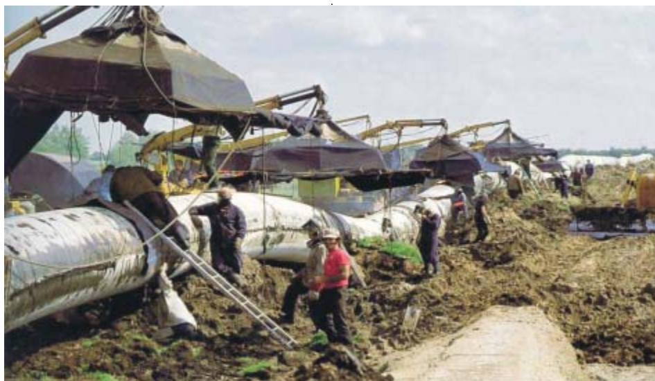
A gas pipe under construction: its energy transport capacity is 50 times higher than an electric transmission line for roughly the same investment.
