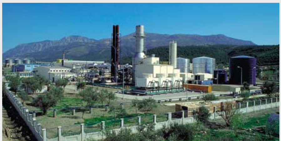
The 54.3 MW baseload plant in Manisa, Turkey, currently powered by three Wärtsilä 18V46 generating sets, will be extended to 84.8 MW.
