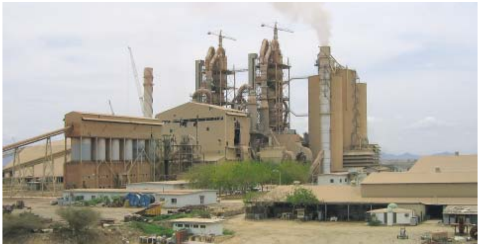
The SPCC cement plant close to Jazan.
