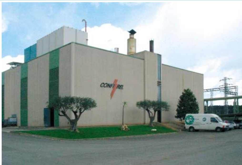
The Confirel power plant of Papelera La Confianza.
